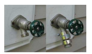
Hose bib with BFP; water supply is protected from contamination when a hose is connected.
